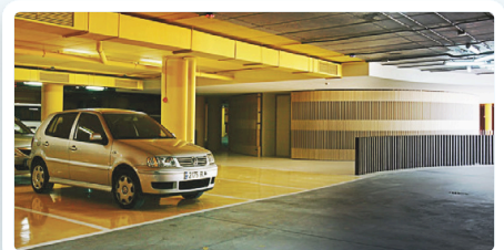
Car Park Floors
