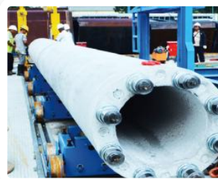
Segment Assembly with Post-tensioning
