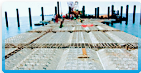
PRECAST HALF SLAB
