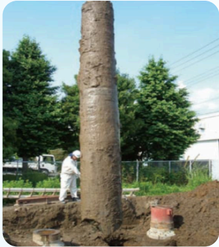
EASE PreBore Method Pile Socket
