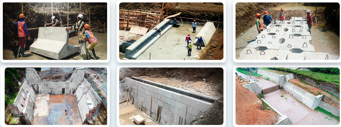
Pilot Project Sabodam Modular, Kediri, East Java
