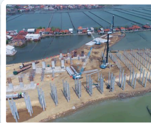
Piles Foundation for Bridges
