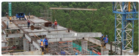
Beam Installation
