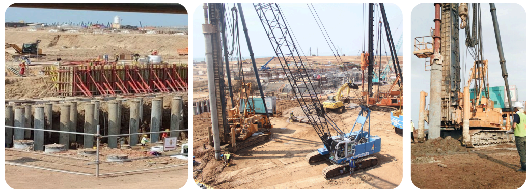
Central Java Power Plant (CJPP), Batang Regency, Central Java Province
