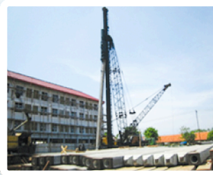
Piles Foundation for Building
