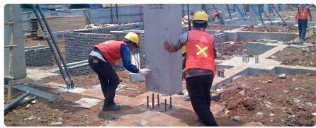
Column Installation
