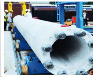
Segment Assembly with Post-tensioning
