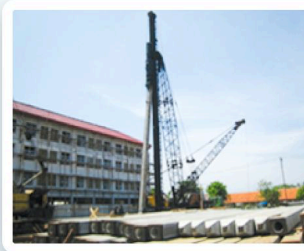
Piles Foundation for Building
