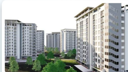
Paspampres Tower Housing – IKN 12 floor ; 10.000 m 2 ; 2 month (Structure works) Precast Column, Beam & Full Slab
