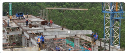
Beam Installation
