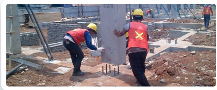
Column Installation
