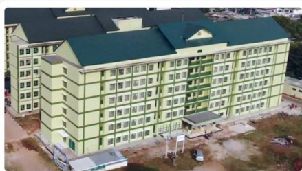
TNI/Polri Tower Housing – Jakarta 6 floor ; 5.000 m 2 ; 3 month (Structure works) Precast Column, Beam & HCS with PRESS System
