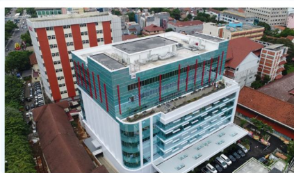
St Carolus Borromeus Hospital – Jakarta 12 floor ; 25.000 m 2 ; 4,5 month (Structure works) Precast PC wall for basement, Column, Beam & HCS with PRESS System
